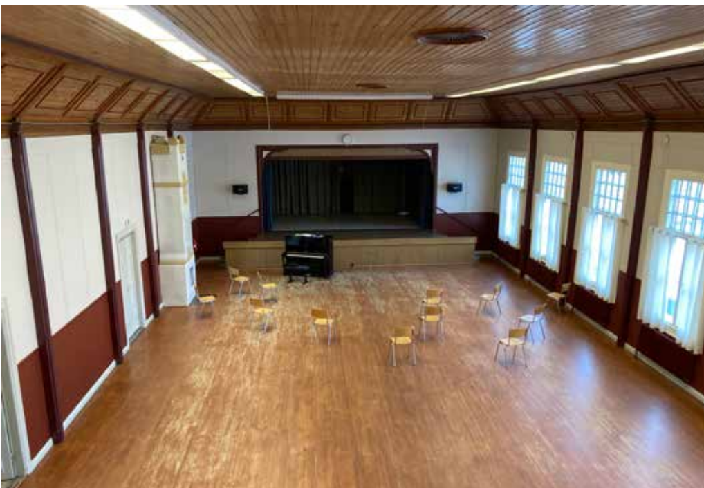
The main hall and the stage. The ceiling has retained its original colours.
