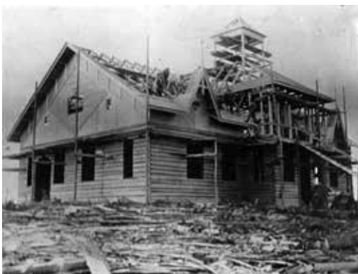
The construction of the labour hall. The Punkalaidun Workers' Association.
