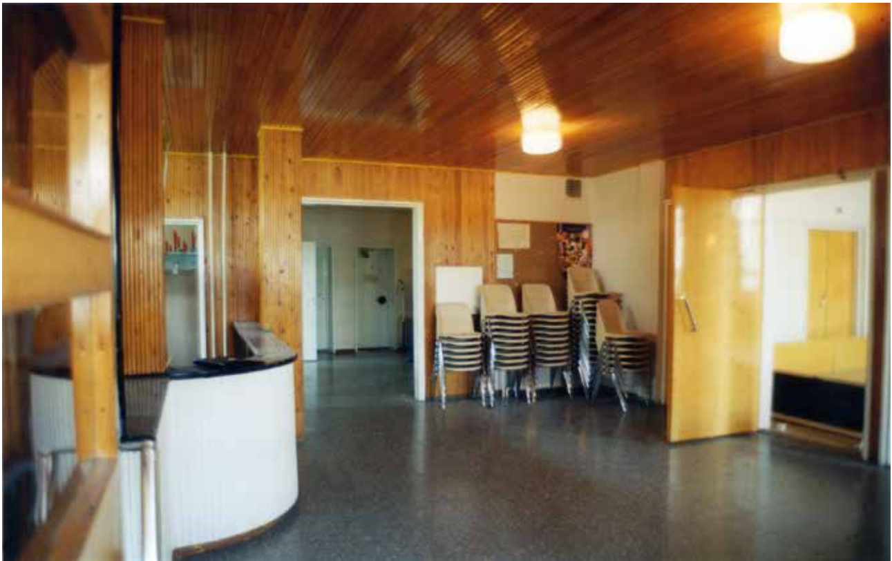
The original finger panels with a lacquer finish and the flush-panel doors are preserved in the lobby. Olli Anttila, The People's Archives.
